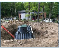
An off grid rural property owner installed 2 x 6500L Carat tanks outfitted with Optimax self-cleaning filter package and a Grundfos SBA-45 pump. The system will collect rainwater from the 900 sq. ft. roof of a new garage building. The water will be used to water landscaping and to supply a wash station in the garage. With 2 tanks the owner installed the filter package in one tank and the pump in the other tank to ensure ease of access for any future pump maintenance.
