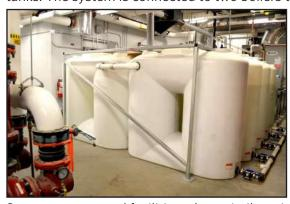
Zamboni ice resurfacing machine. The full tanks, installed in the warm mechanical room, also absorb the ambient heat that helps to warm the water prior to entering the boilers therefore saving energy on heating the water. Global Spectrum's Dan Rubino, (the facility operator) Director of Special Projects said the company is looking at other possible Global
