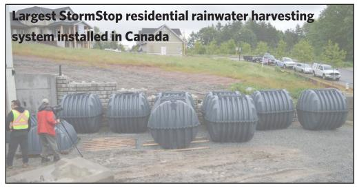
As part of the R-2000 Net Zero Energy Home pilot project by Natural Resources Canada, SonBuilt Custom Homes Ltd, and University Sprinklers have successfully installed the largest residential GRAF rainwater harvesting system in Canada. The nine 1,700 US gallon GRAF Carat tanks from BARR were installed belowground, connected together for a maximum storage capacity of 15,300
